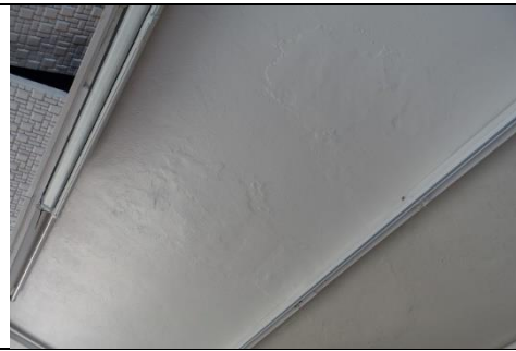
Figure 58 – Damp damage to plaster ceiling over stage in function room. (Source NBRSArchitecture, March 2018)
