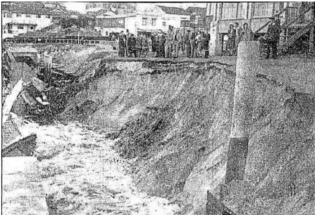
Figure 17 — Collapsed seawall, kiosk and surf pavilion at North Cronulla. (Source: 'Council will Abandon Clubhouse to the Sea', The Sun , 25 August 1946, p.1.)
