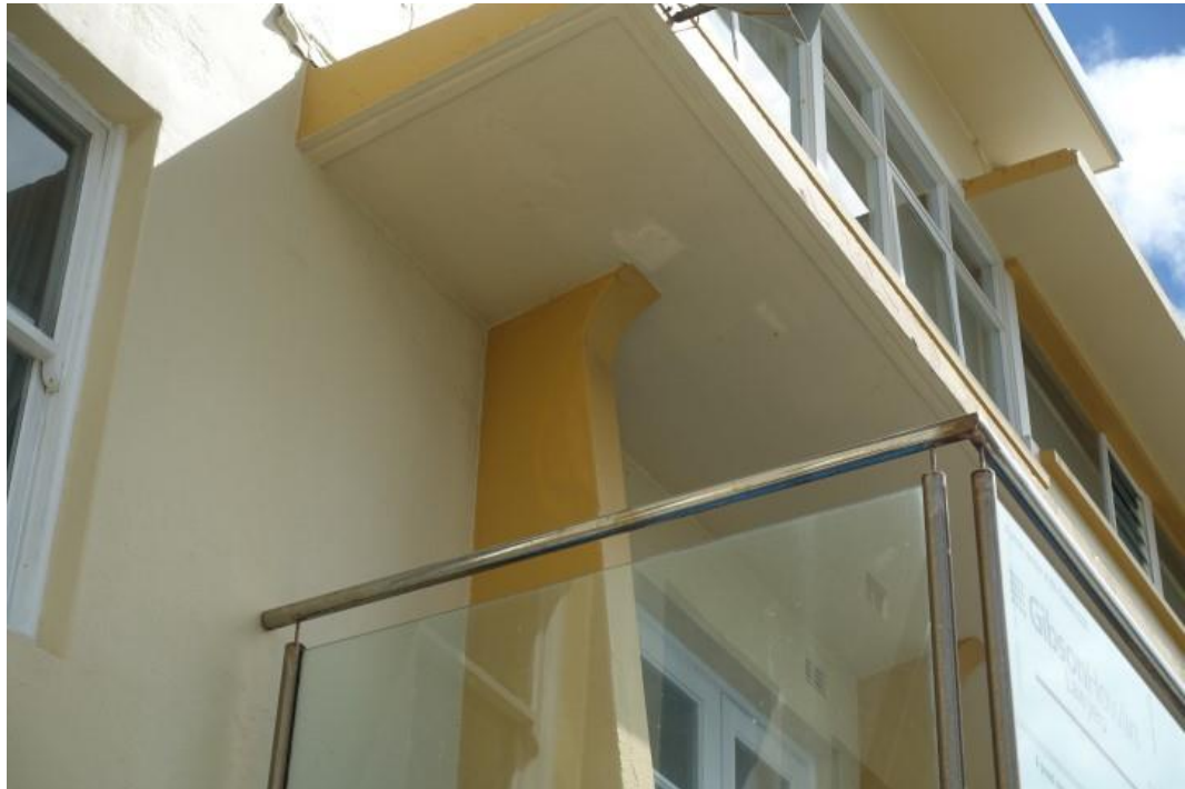
Figure 47 – Detail of reinforced concrete balcony and sunshade on east elevation. (Source NBRSArchitecture, March 2018)
